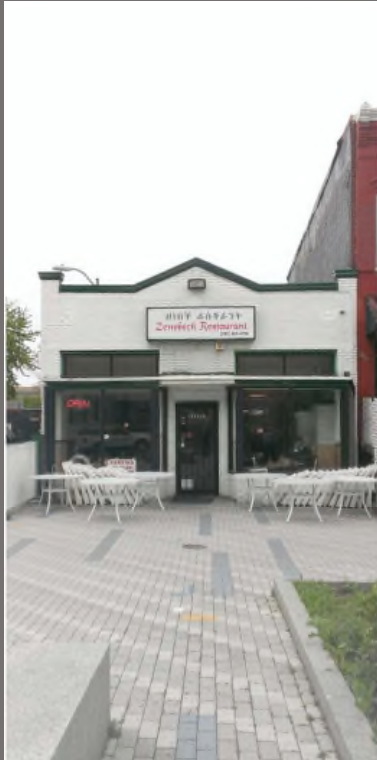
608 T St. NW Lot 35 To Be Demolished
