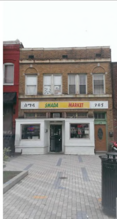
614 T St. NW Lot 33 To Be Demolished
