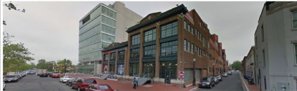
3 - S STREET LOOKING NORTH DOWN WILTBERGER STREET
